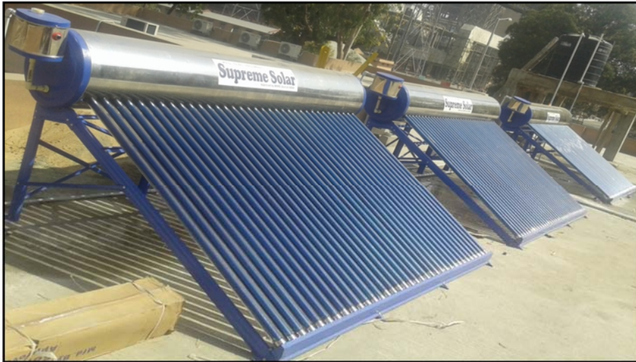
Solar Water Heater at Plant
